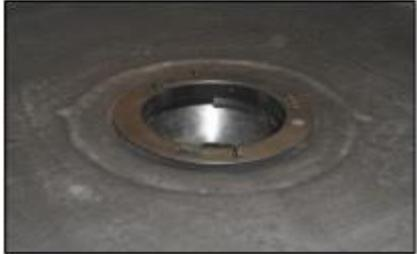
6) Screw in the clamping ring till it's completely tightened. Use the two tightening lugs to apply leverage to the ring. Once tight the membrane should be visibly pulled into the outlet.
