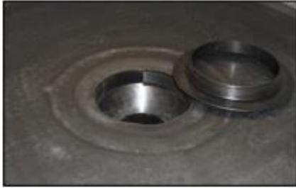
5) Ensure the membrane is clean and the outlet is free of any debris.
