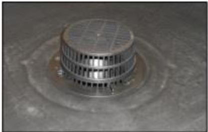
7) Install the leaf grate into the three locating tabs.
