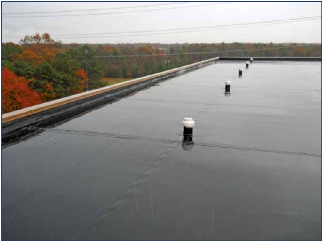
Figure 8 – One-way air vents installed along edge of disbonded EPDM membrane area.
